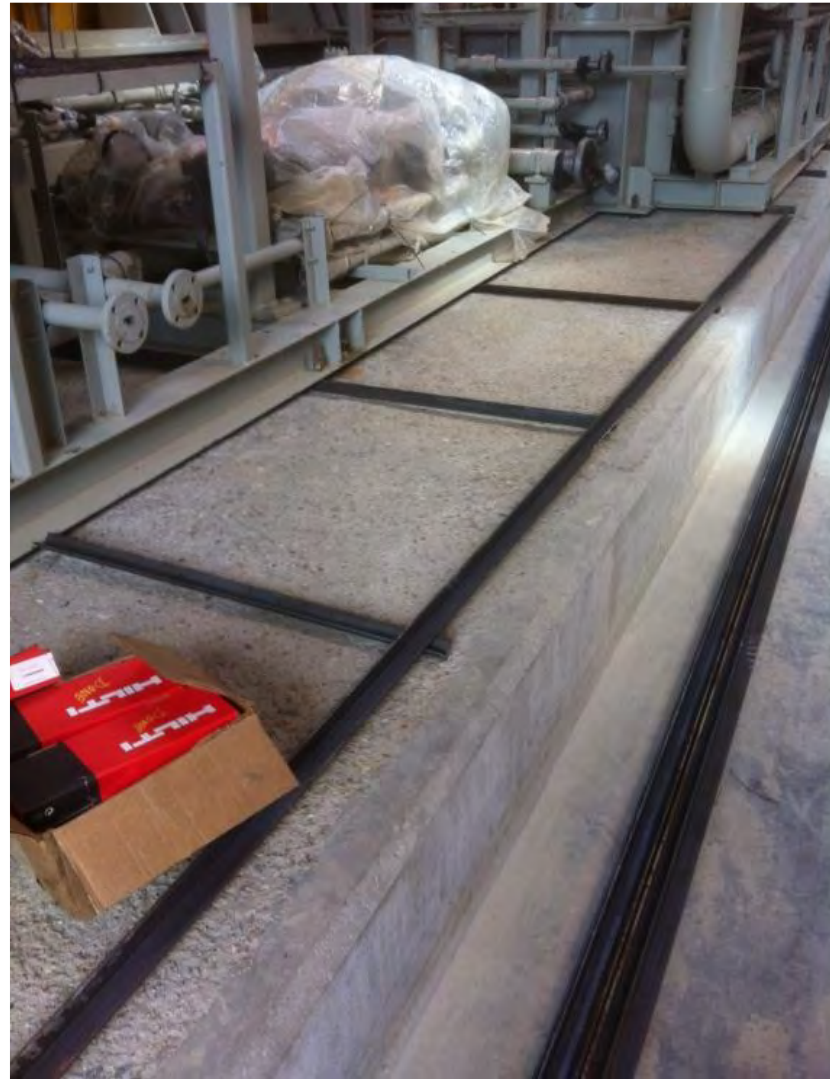
Joint placements made before the skid is set.
