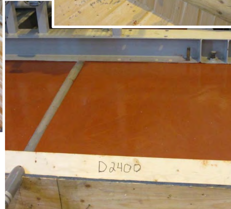
In-situ (pumped) joints
